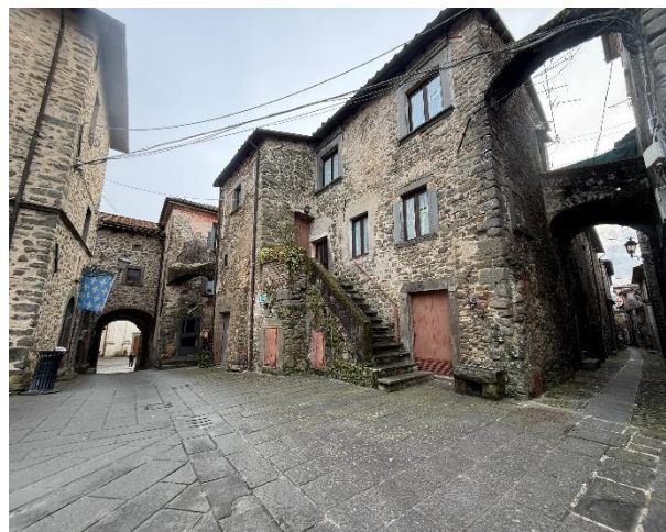
Figure 11 arch to the left of Piazza del Pozzo with ramp greater than 8%
