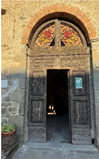
Figure 26 entrance to unequipped toilets
